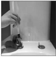
4. Lock the support completely on the ceramics and cover with stainless steel cover.
