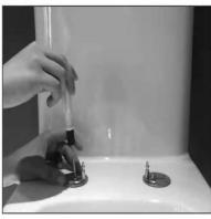
2. Tighten the setscrew but not to the end in order to adjust the seat cover properly.
